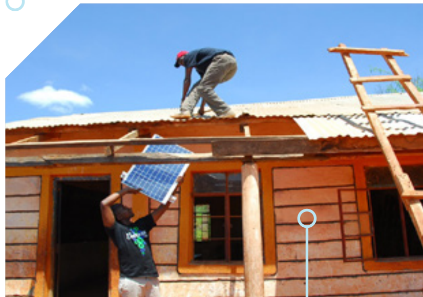
IEEE's Kenya student branch installs solar panels at the isolated Kasiluni Primary School, the only institution of its kind within a 25-kilometer radius. The school serves 600 pupils in six grade levels.
